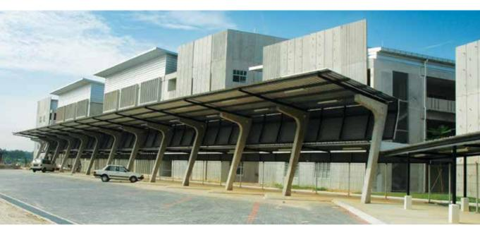
The best comfort in this complex is the passive solar sun shading skin that wraps around the external envelope. It gives even reflective light throughout the day with cool winds cross ventilating through adjustable louvres. A complex system of rainwater harvesting is put in place where most of the skillion roofs' water are channeled
